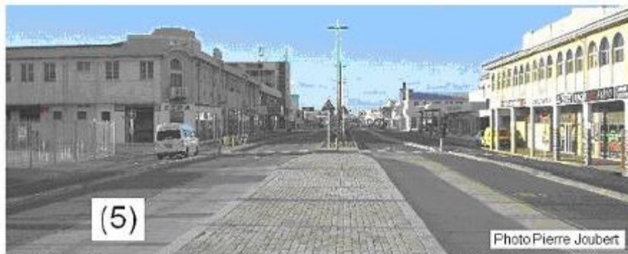
Throttling of general traffic lanes. Typical section of NMM BRT in narrow Govan Mbeki - two bus stops next to each other use up 5 lanes of road space, leaves only two for general traffic and no parking for business.
