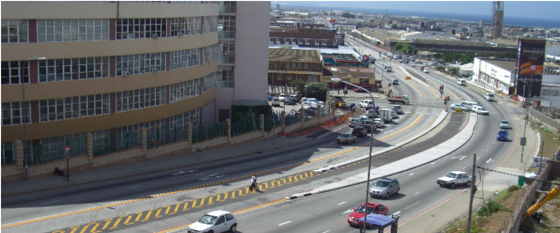
1. Section between Standford Road and CJ Langenhoven after completion in 2011
