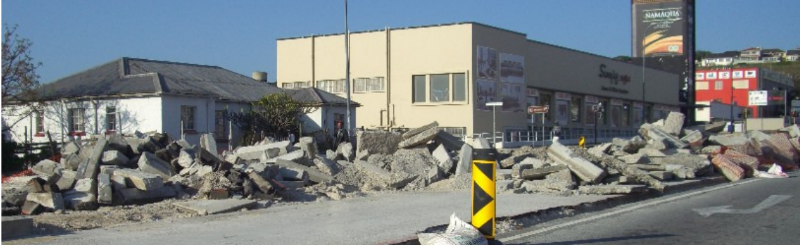
3. Large amount of material removed during demolition phase
